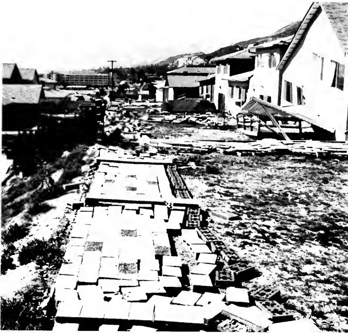
Photo 17. Example of garden wall failure (Almetz Street-Aldergrove Avenue). Note Olive View Hospital in background. Courtesy of Charles A. Yelverton.
